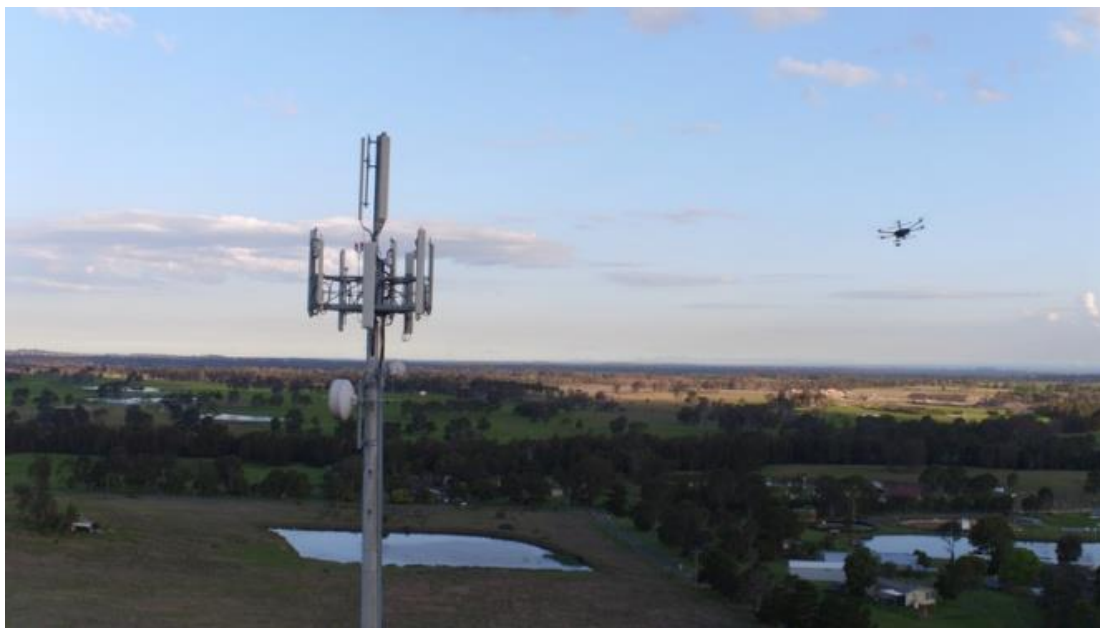
Fig 5.3.7: Cell tower inspection using drone
